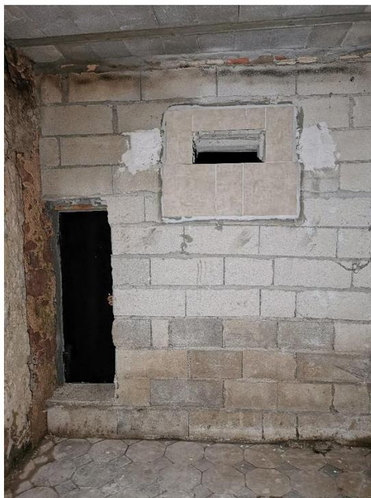
**PHOTO 4 : ACCES A LA CAGE D'ESCALIERS – PORTE METALLIQUE – OUVERTURE POUR LES CHAUVES-SOURIS ENTOUREE DE CARREAUX DE FAIENCE**
